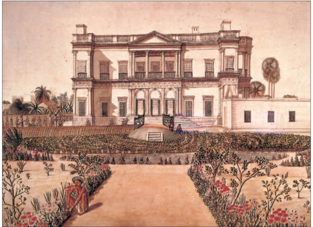
As the British began to establish themselves in India, they imported their own architectural styles, as shown in a watercolor of a house built at Chapra in 1796.
