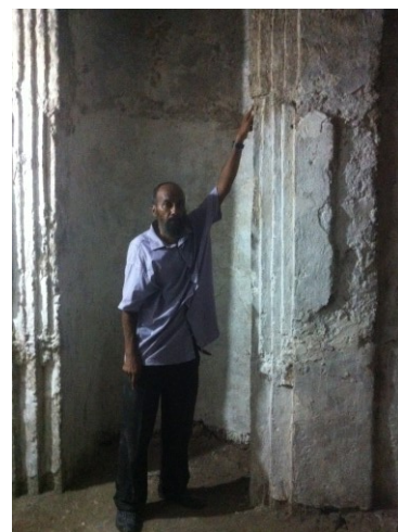
Fig. 6. Underground of Sharif Ahmed Mosque. The Two mihrabs of the ancient buried mosques.
