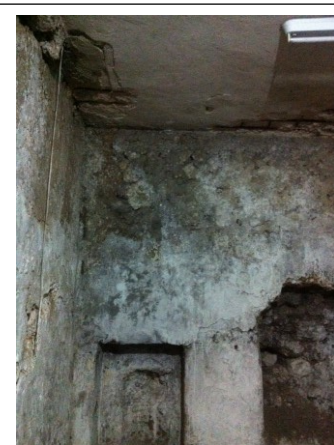
Fig. 8. The niches of the ancient underground section of Sharif Ahmed Mosque. The need for their repairing is evident.
